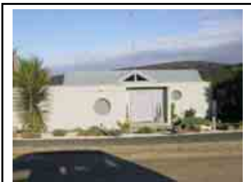
Lack of setback increases a building's prominence
