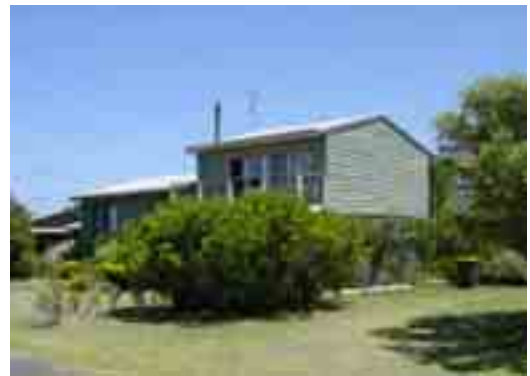
Timber cladding and colourbond roof characteristic of housing in the Study area
