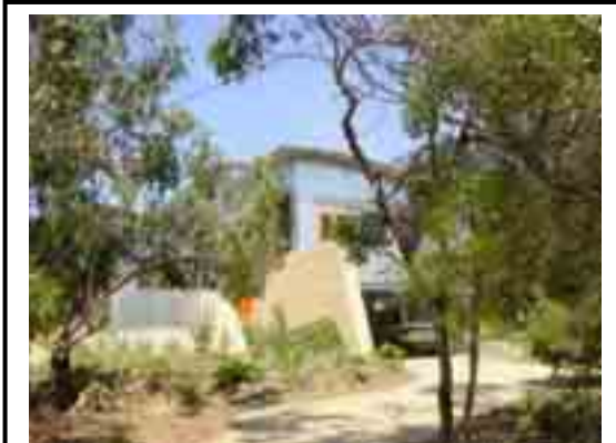
Setbacks generally provide for vegetation that screens buildings in part from the street
