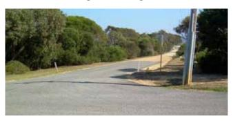
Further correspondence with another council officer stated that intersections were sealed as a matter of safety, and that the sealing was spray seal, considered to be a short-term solution envisaged to last not more than five years. The question then is what happens when the spray seal breaks down? Will the residents be left with an unsightly mess of pot holes at that intersection?
