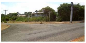
Further, the sealing of only 50 metres from the intersection creates an unstable interface between the sealed and unsealed sections. It is here that the road surface is most vulnerable, resulting in degradation of the surface, and dangerous driving conditions.
