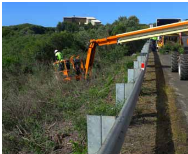
Cutting and removing woody weeds with the aid of a knuckle boom machine (Mad Max house in background)
